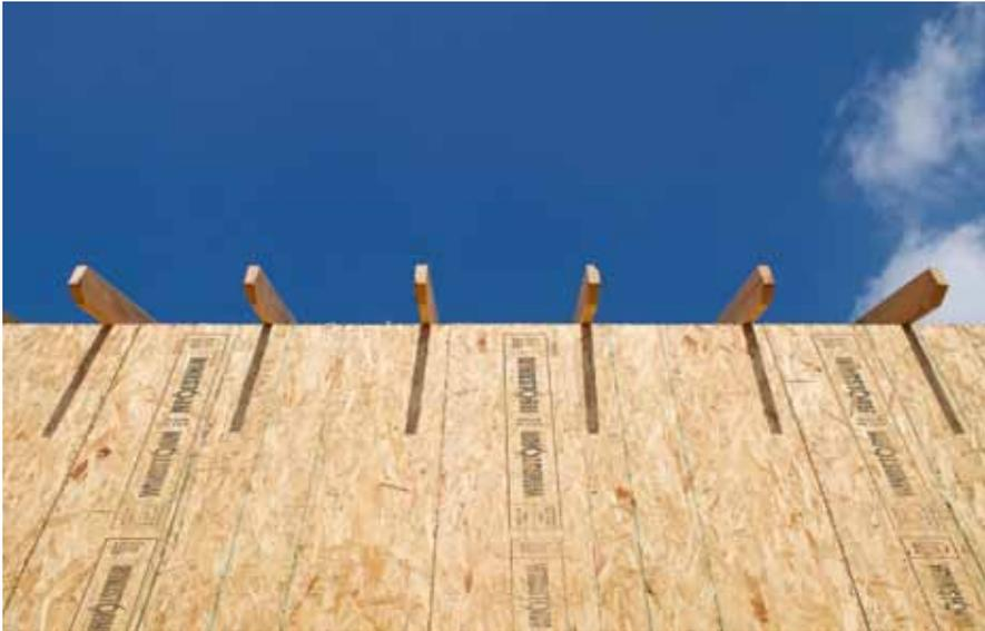
Tests conducted at Virginia Tech University showed that 4x10 TallWall OSB sheathing installed vertically and spanning from top plates into the joist area increased the overall strength of a 9-foot-high wall by 38 percent compared with the same wall sheathed with 4x8 OSB panels.
