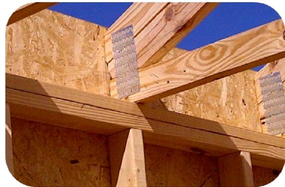
*When used with raised heel trusses, TallWall and Windstorm sheathing allows full depth attic insulation to the outside edge of the top plate.*
